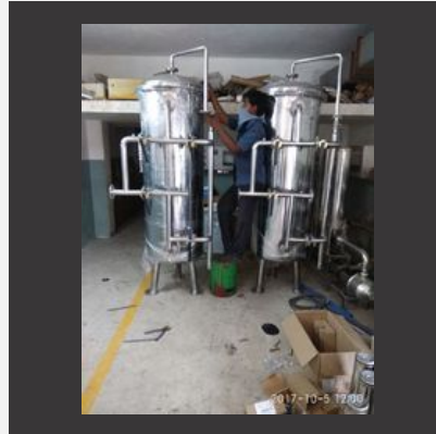
Stainless Steel Fabrication Work
